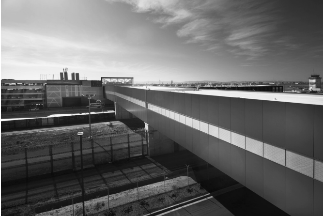
Above: An informal taco shop built in the front yard of a Victorian home in a San Diego mid-city immigrant neighborhood. Courtesy of Estudio Teddy Cruz + Forman. Below: Cross Border Express in Otay Mesa, California. Photograph by Harrison Photographic.
