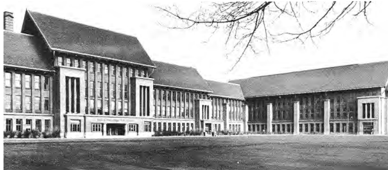
Carl Schurz High School, Chicago, 1910 by Dwight Perkins displayed no ornament or historical eclecticism and is perhaps the earliest example of open-planning in schools where parts of the same school are differentiated to house various activities. 22
