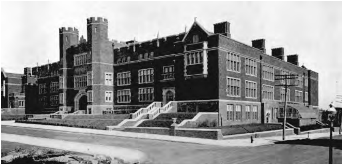
Figure 3.4 Grover Cleveland High School in St. Louis, Missouri 1921. 17 Note windows on all facades admit natural light.
