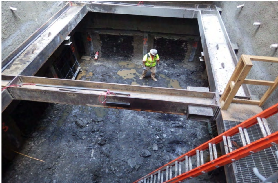
Figure 15: Installation of Third Strut and Waler at 48-ft below ground surface (Photos by Parsons Brinkerhoff [2]: Jan-2014)
