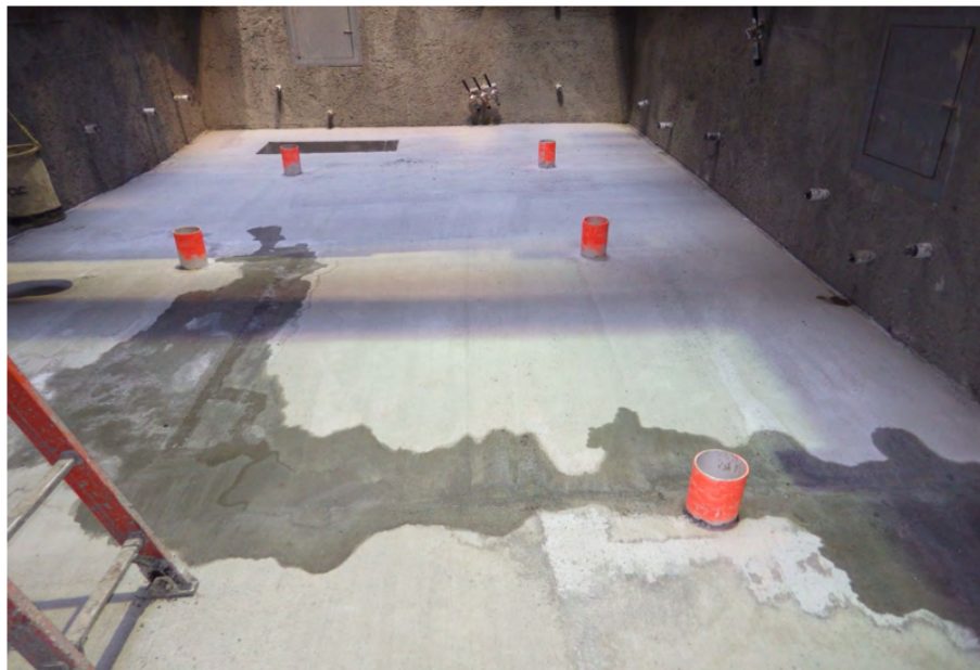
Figure 17: Installation of Invert Slab at 72.5-ft below ground surface (Photos by Parsons Brinkerhoff [2]: March-2014)
