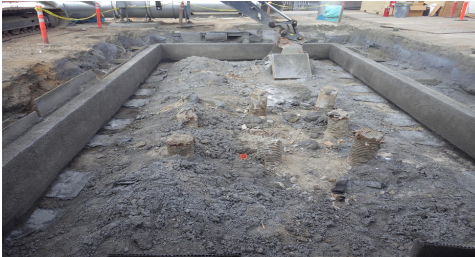
Figure 12: Excavation to 5-ft within Exploratory shaft, Installation of Cap Beam (Photos by Parsons Brinkerhoff [2]: Sept-2013)
