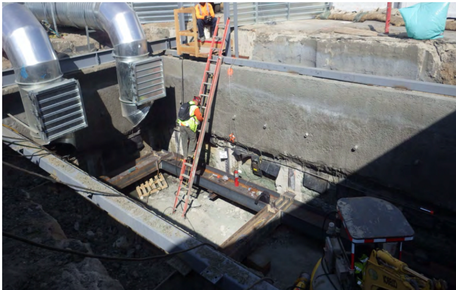
Figure 13: Installation of First Strut and Waler at 15-ft below ground surface (Photos by Parsons Brinkerhoff [2]: Oct-2013)
