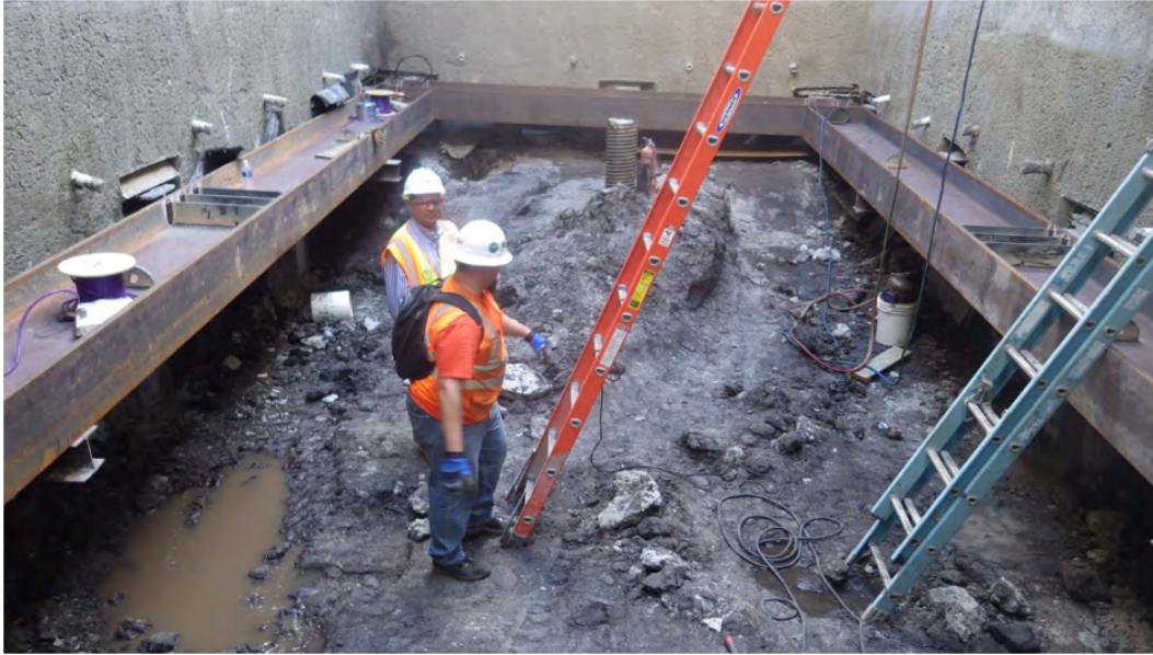
Figure 14: Installation of Second Waler at 29-ft below ground surface (Photos by Parsons Brinkerhoff [2]: -2013)
