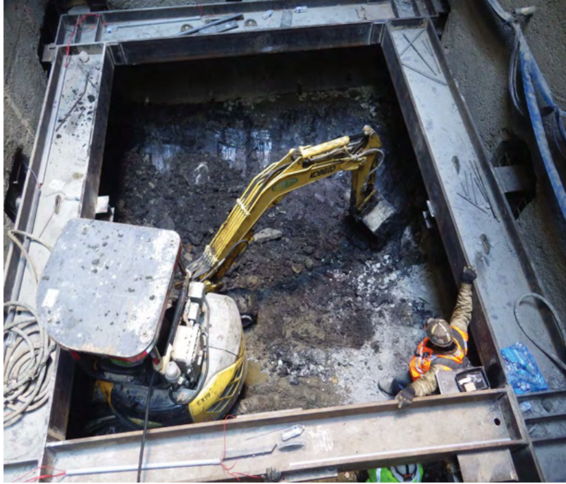
Figure 16: Installation of Fourth Strut and Waler at 63-ft below ground surface (Photos by Parsons Brinkerhoff [2]: Feb-2014)
