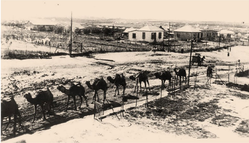
Figure 3. Camels carrying crushed seashells ( zifzif ) for construction in Ra'anana, mid-1920s (Ra'anana Municipal Archives).
