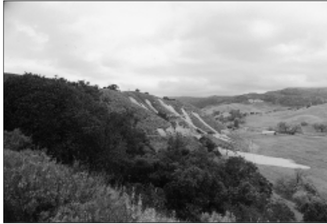
A side view of the same impressive landslide that appears on page 1. Photo by Patti Parisi
