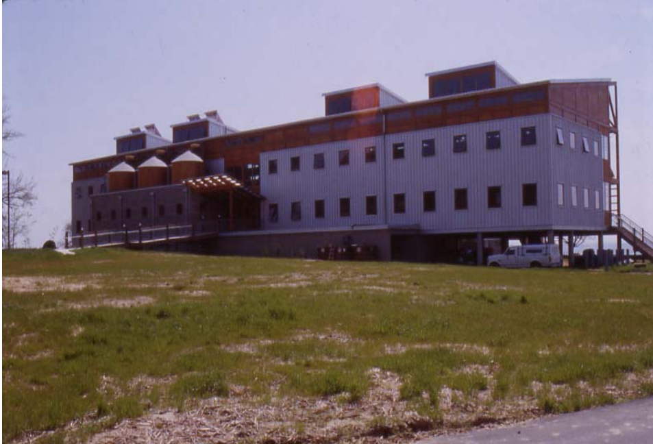
Photo 1. Entry side of the Philip Merrill Center Building shows the rain water capture system in the round towers.
