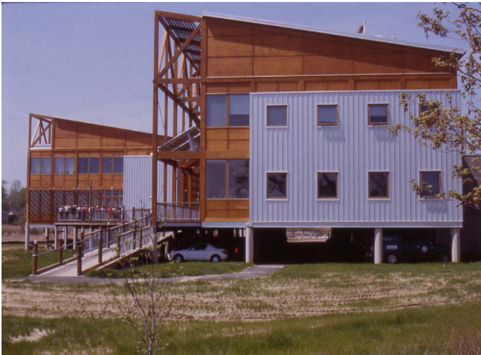
Photo 2. East side of the building with the Conference Center and outdoor deck on the far left. Shading devices on the south side of the building enclose an external walkway. Photo voltaic arrays can be seen on the sloped part of the shading device.
