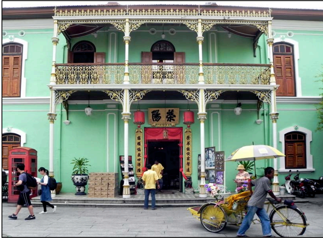
Figure 5. The exterior of the Pinang Peranakan Mansion, featuring European iron latticework. Source: Hajotthu (2010). Licensed under Creative Commons.
