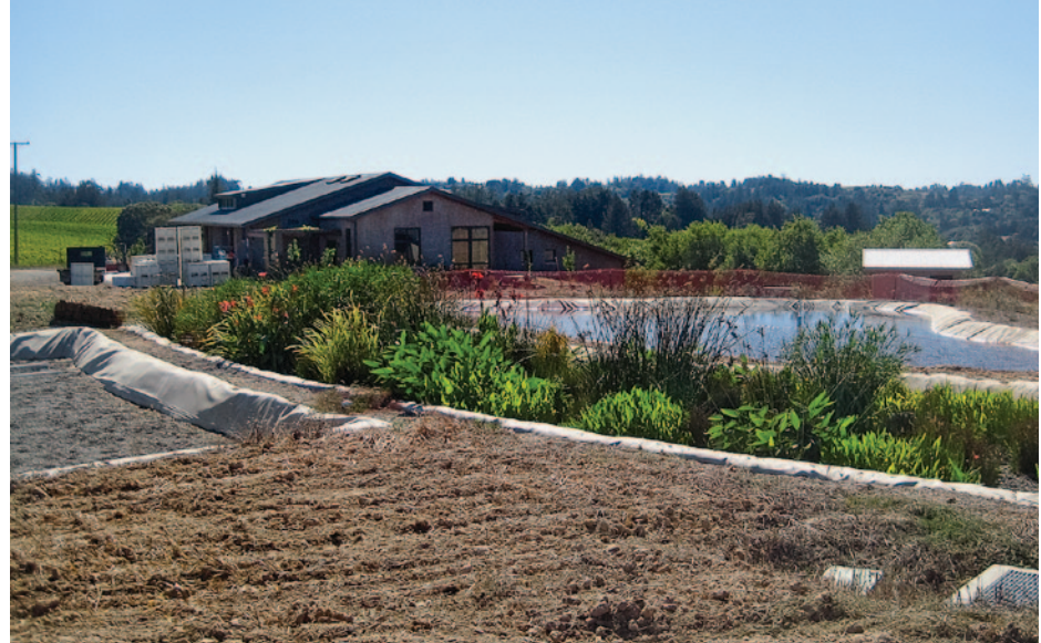
Natural treatment systems are effective in reducing organic-matter levels in wastewater, and even more so when they incorporate plants. At Lemon Winery in Sebastopol, constructed wetlands include a planted bed (center) and an unplanted pond (middle right).
