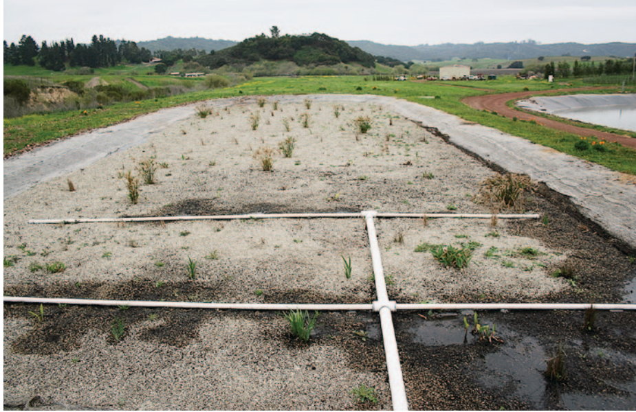
Piping disperses process wastewater across the width of a constructed wetland at a Paso Robles winery. Samples were taken at the outflow (not shown) and the far end of the wetland, which was designed to handle wastewater generated by producing 14,000 cases of wine.
