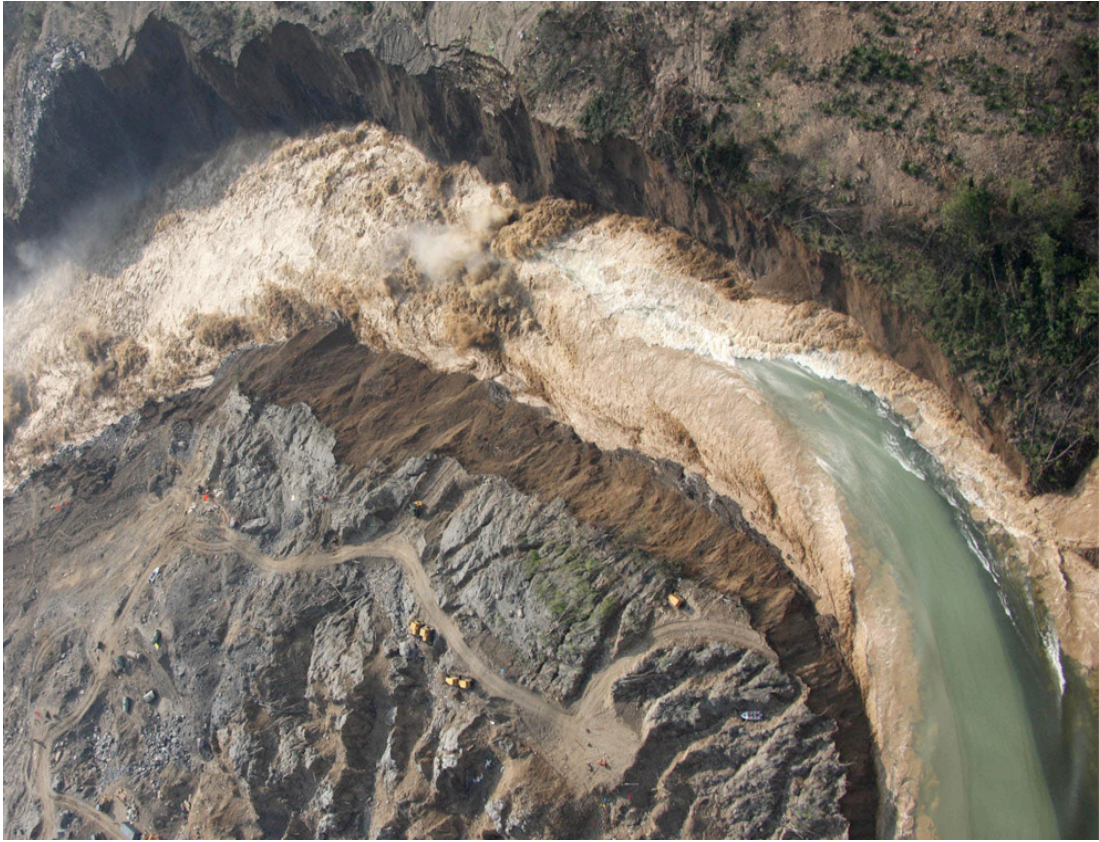
Figure 16. The release of Tangjiashan Lake and the resulting riverbank erosion.
