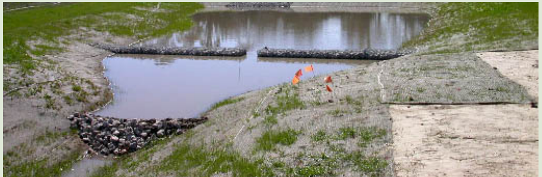
Water retention in the storm water management system following the first winter rains.
