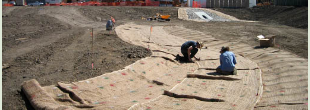
CCBER staff installing coconut netting for erosion control in the storm water management system.
