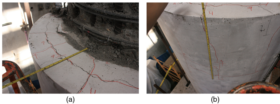
Fig. 7. Damage in the pile of Specimen 1: (a) circular and splitting cracks; (b) lengths of splitting cracks
