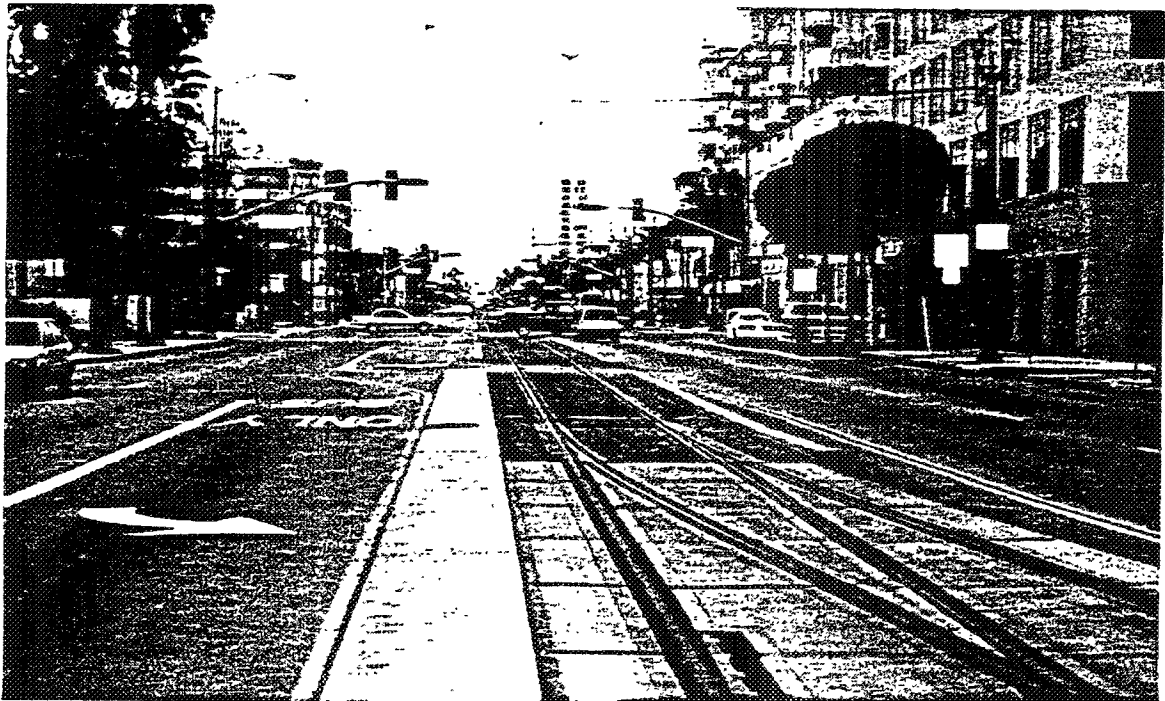
Photo Series 4.32 Transit Mall station: North view of Pacific Avenue in the station area. Residential activities are limited to condominiums and apartment buildings, some of which can be seen to the right hand side of the photo.
