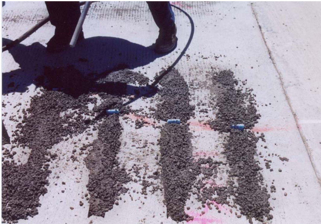
Figure 2.24. Vibration of backfill grout with small stinger.
