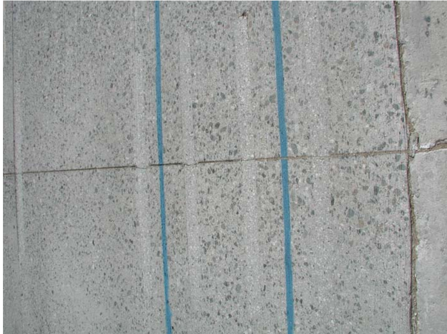
Figure 6.3. HVS Test Section 556FD, Joint 38, prior to HVS testing.
