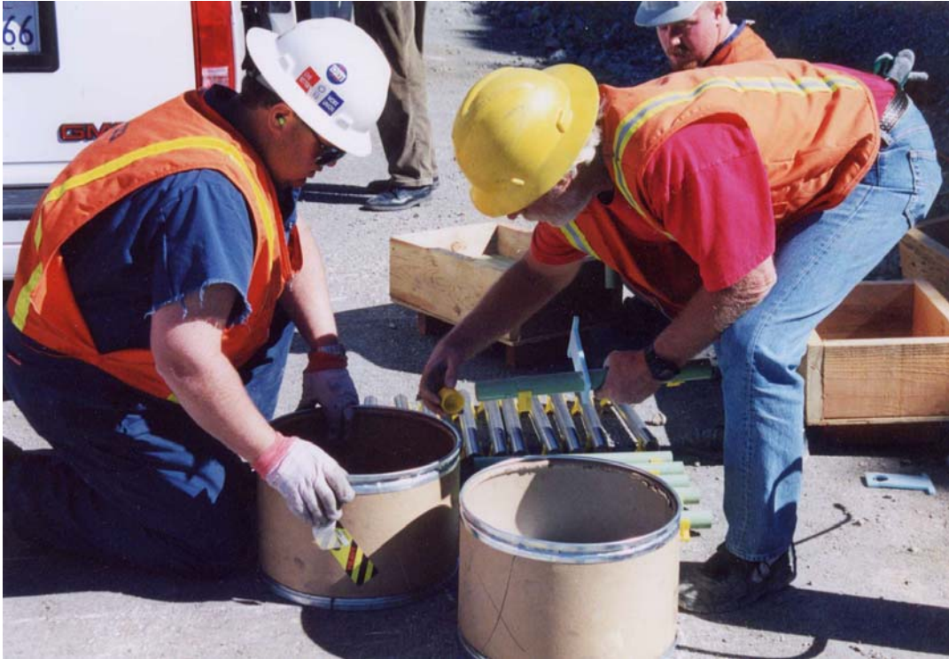
Figure 2.15. Putting together dowel bar retrofit assemblies.
