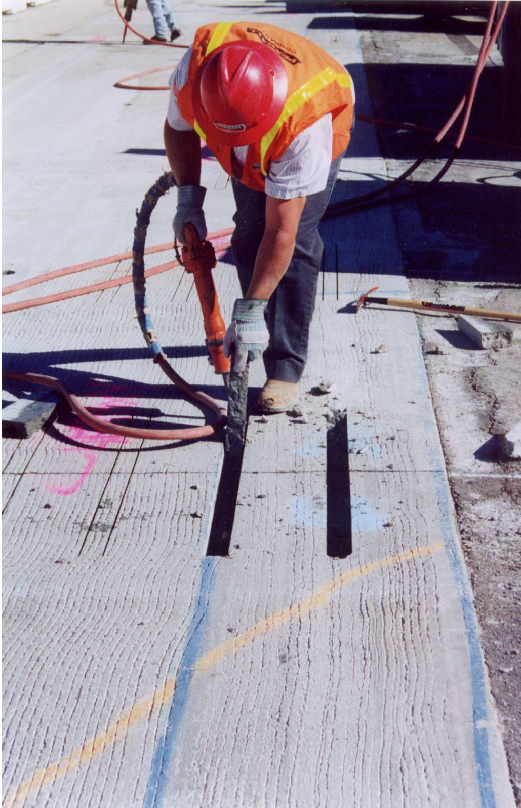
Figure 2.12. Removal of concrete from dowel bar slots.
