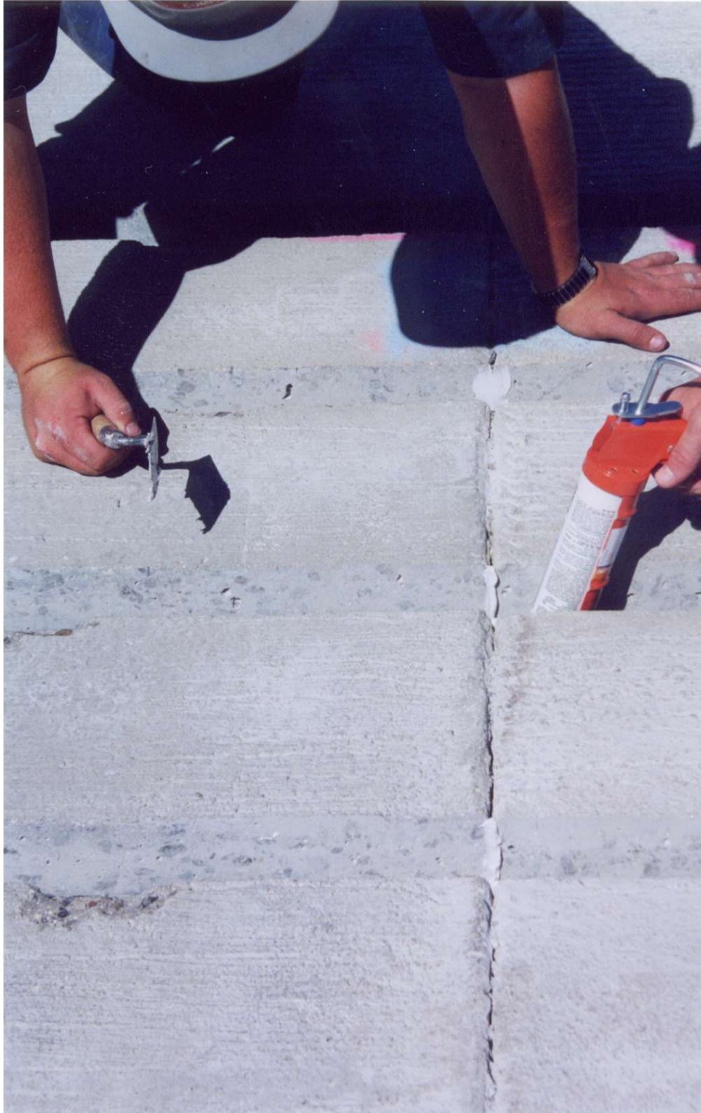
Figure 2.14. Sealing joints with caulk.
