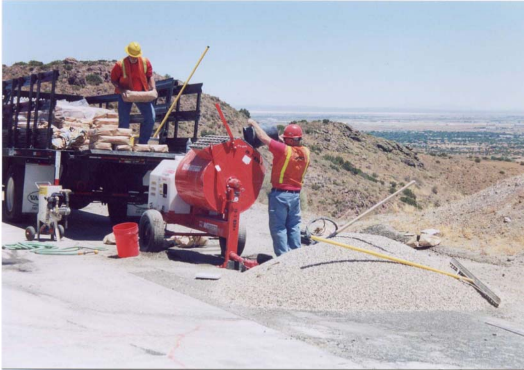
Figure 2.21. Batching backfill grout material into mixer.
