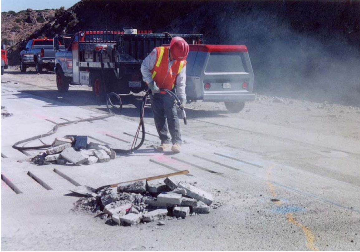
Figure 2.13. Cleaning dowel bar slots with air hose.
