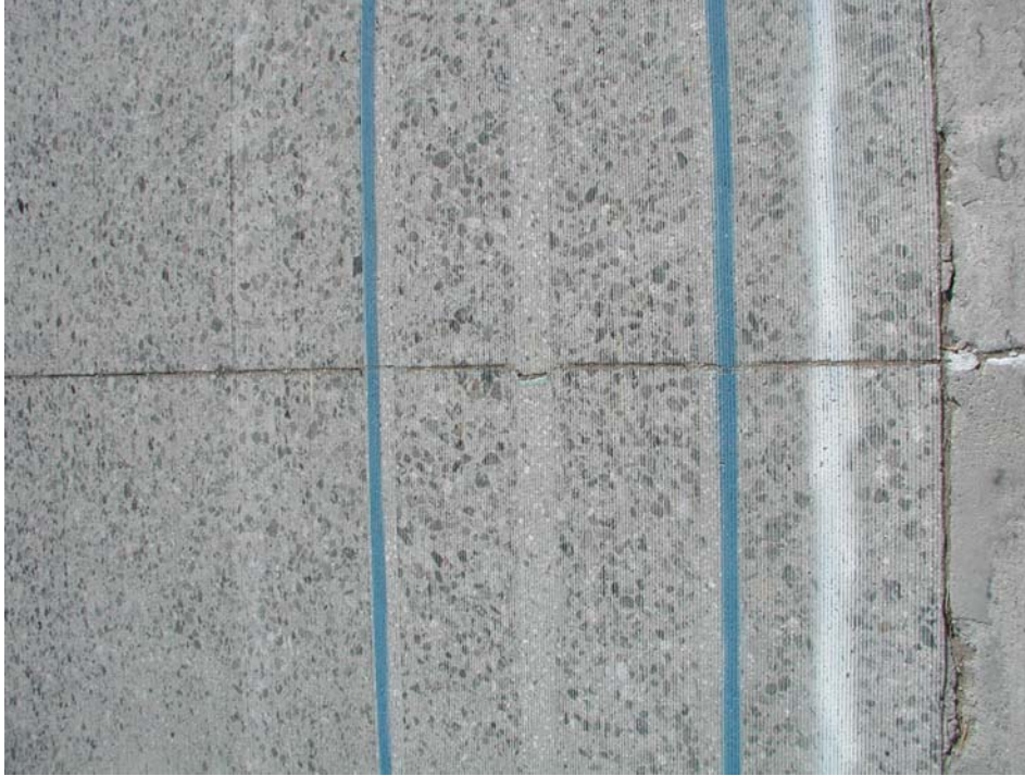
Figure 2.35. Photograph of Joint 36, Section 557FD, in March 2002, showing generally good condition.
