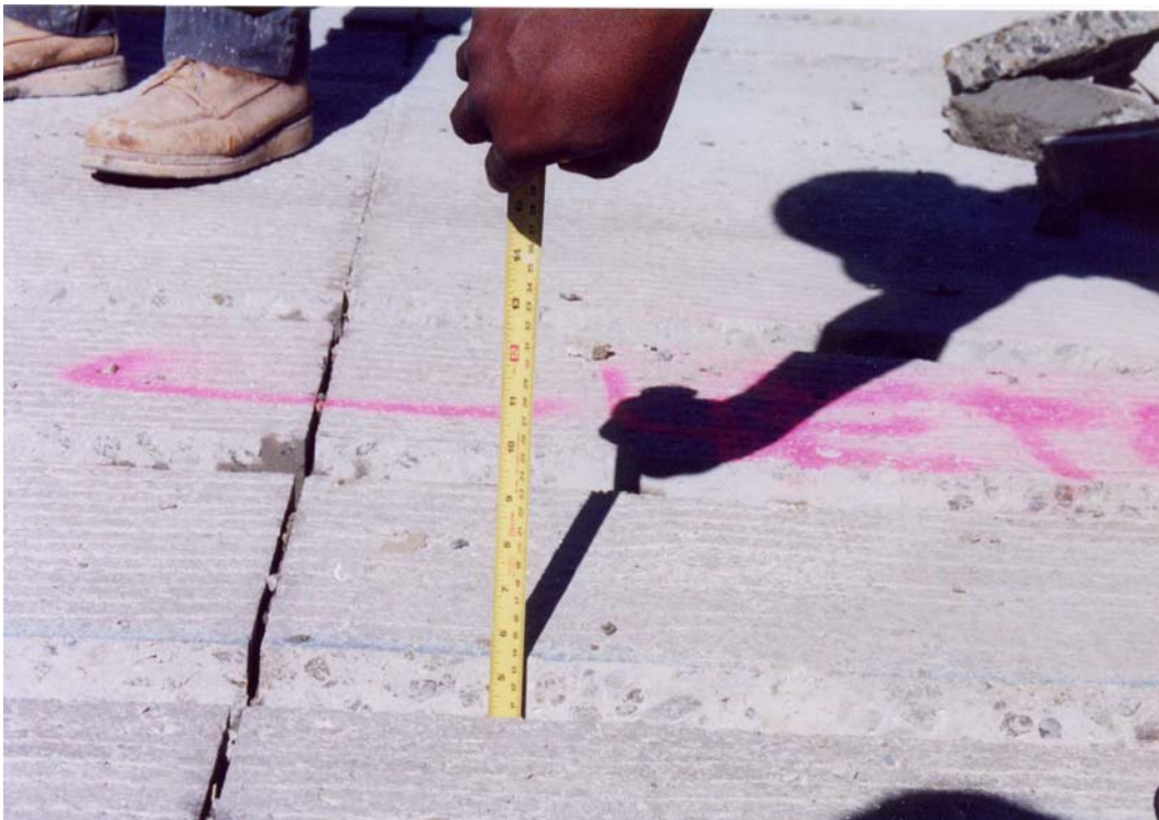
Figure 2.20. Checking dowel bar depth and uniformity of depth.
