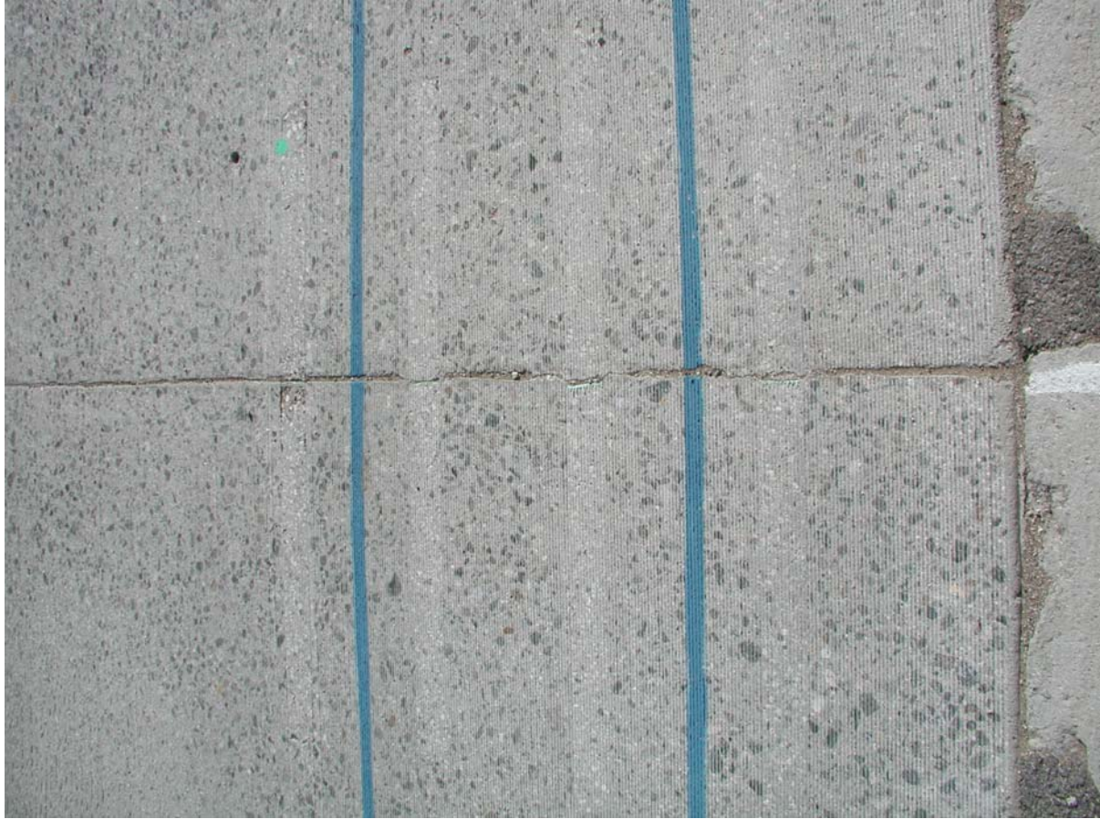
Figure 6.79. HVS Test Section 559FD, Joint 33, prior to HVS testing.
