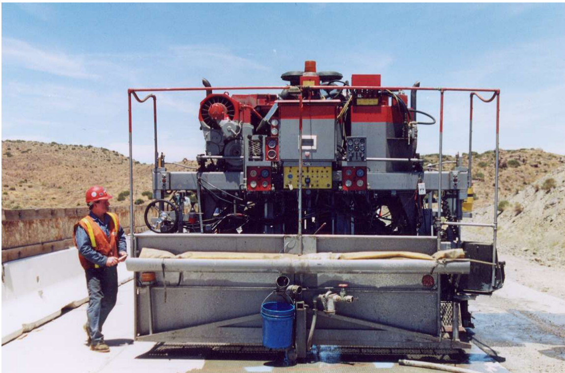
Figure 2.7. Dowel bar slot cutting machine (rear view).
