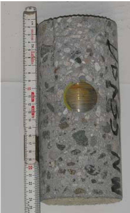
Figure 2.31. Core DBR33NW with epoxy-coated steel dowel located 12 mm above mid-depth of slab.
