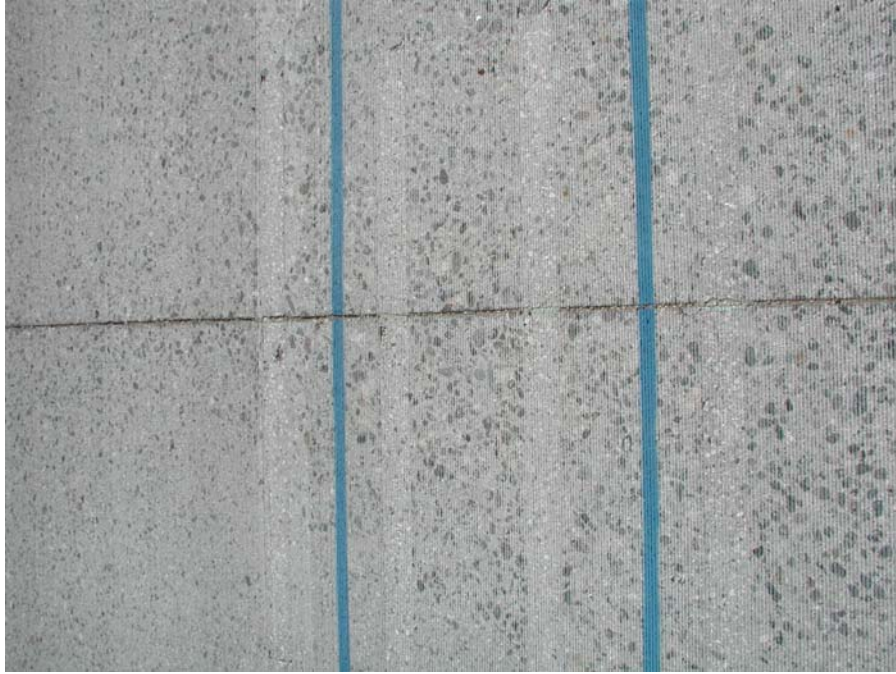
Figure 6.77. HVS Test Section 559FD, Joint 32, prior to HVS testing.
