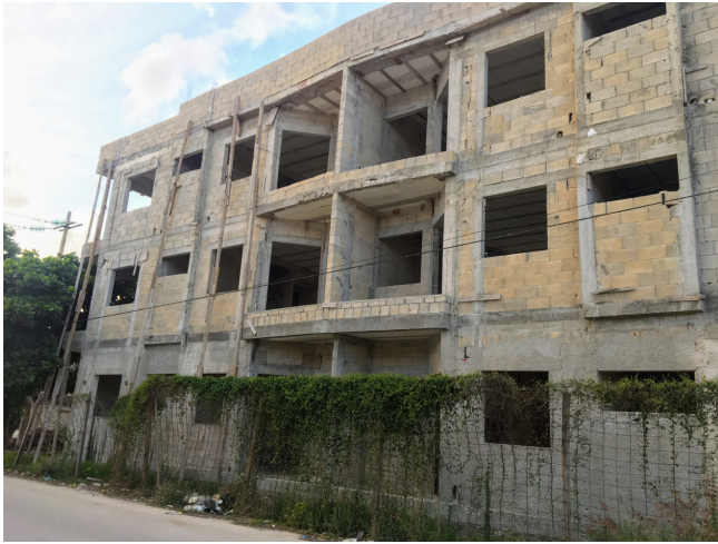
Figure 5. (left) Construction in Tulum pueblo, January 2017
