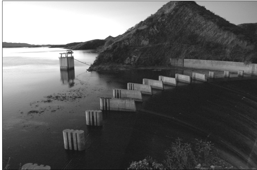
FIGURE 5. Orós Reservoir and Spillway
