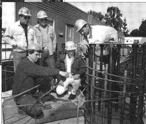
The inspection team is on hand to inspect the steel reinforcing caissons that will provide seismic support for Bldg 90.
