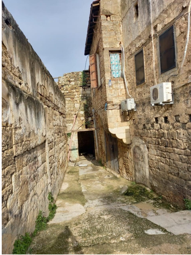
Figure 8. The former entrance to the synagogue (in the center of the image) in the Tripoli neighborhood of Zahrieh. The site has functioned as a tannery and dye factory for over half a decade. To the left of the entrance is the wall of the adjacent Greek Orthodox church. Photo courtesy of Nagi Zeidan. February 20, 2022.
