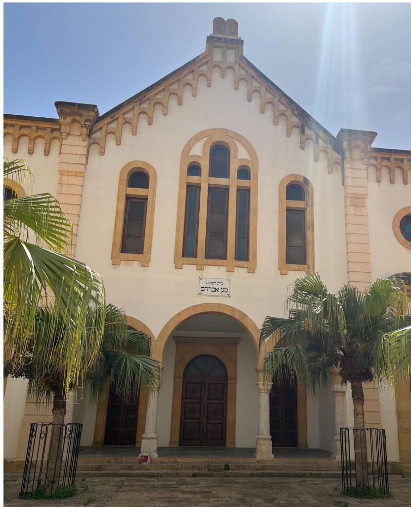
Figure 1. The renovated exterior of Magen Avraham Synagogue in Wadi Abu Jamil, Beirut. Photo © Molly Theodora Oringer (all images are by the author unless otherwise stated), March 24, 2023.
