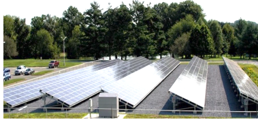
526 527 Fig. 15 NIST-ground array with 1152 PV modules yielding 271 kW. The operation and environmental data from this 528 array are used to evaluate PVPRO.
