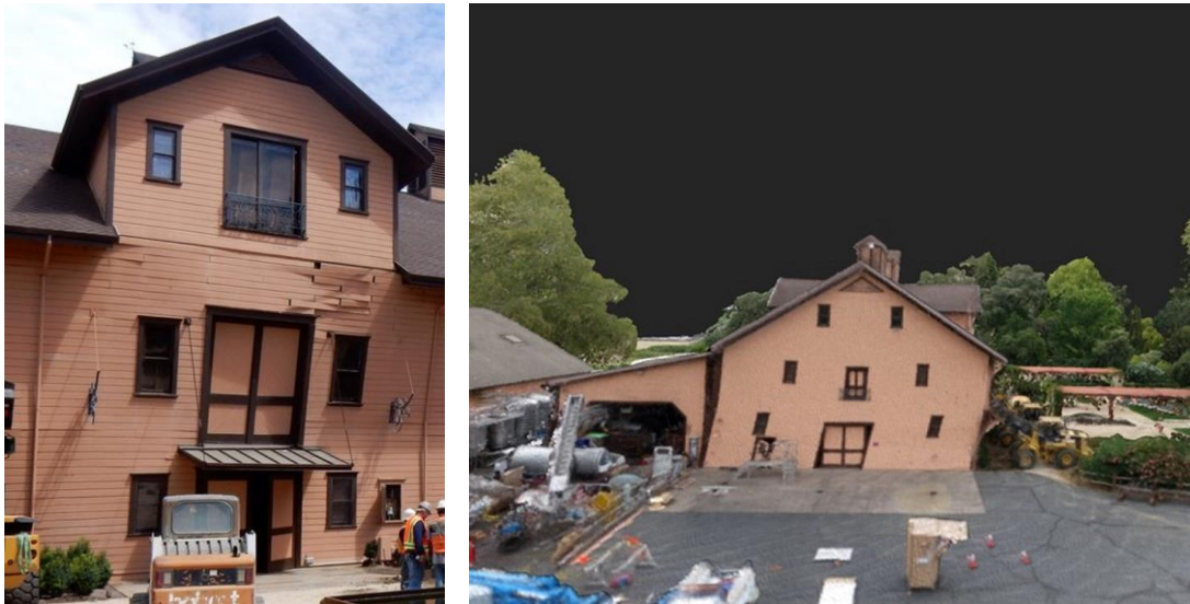
Figure 3.16 Photograph (left) and SfM point cloud (right) of the damaged vineyard structure.
