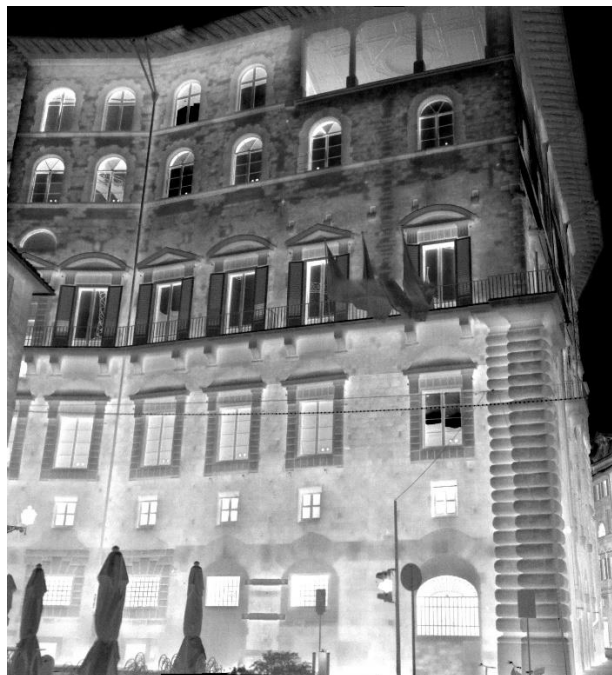
Figure A.1 High-resolution thermal image mosaic of South Exterior wall of Palazzo Vecchio.
