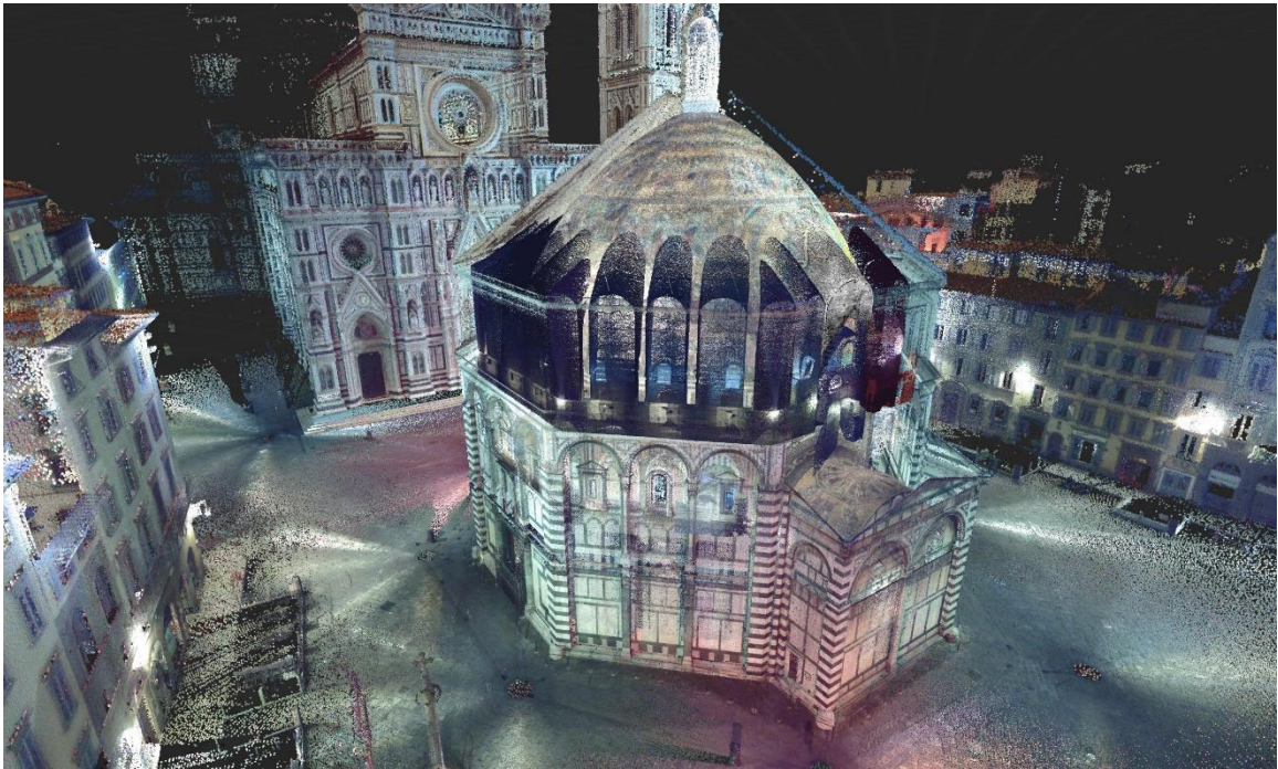
Figure 3.5 TLS data set for the Baptistery di San Giovanni showing the surrounding structures as well as the internal dual shell construction.
