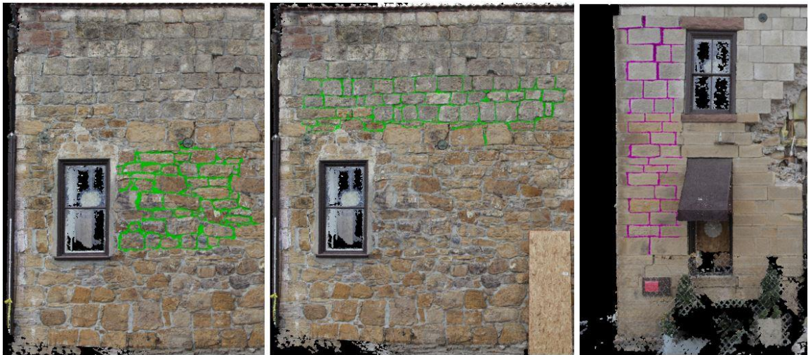
Figure 3.21 Semi-automated annotation of mortar joints.
