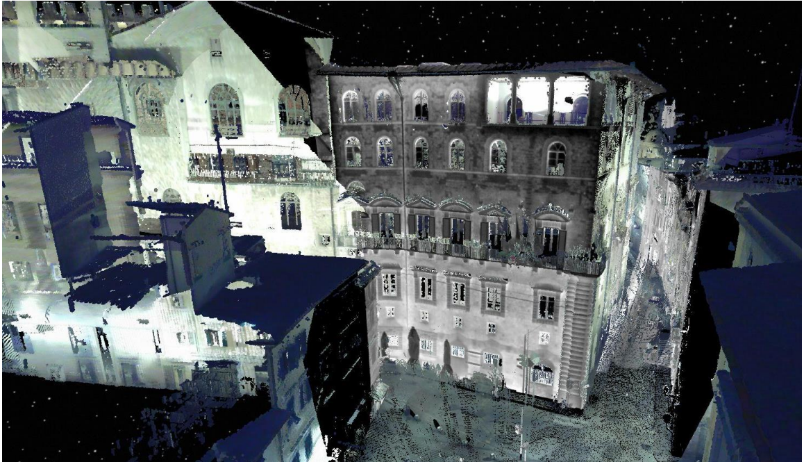
Figure A.4 Thermal image projected onto the geometry of Palazzo Vecchio to enable inspection and measurement.
