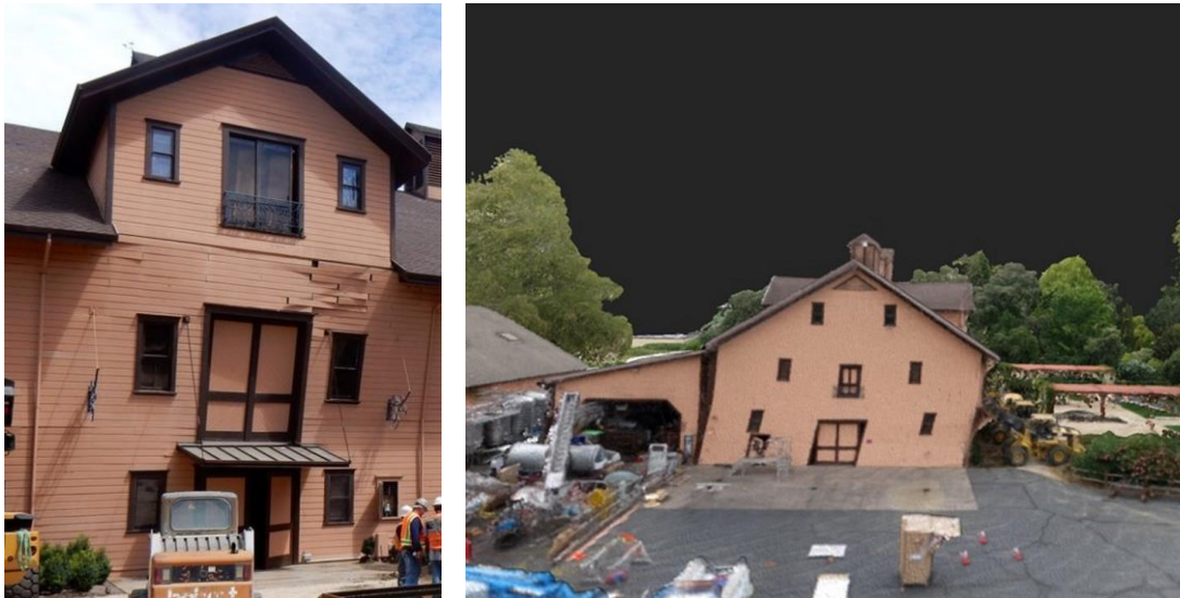
Figure 3.16 Photograph (left) and SfM point cloud (right) of the damaged vineyard structure.
