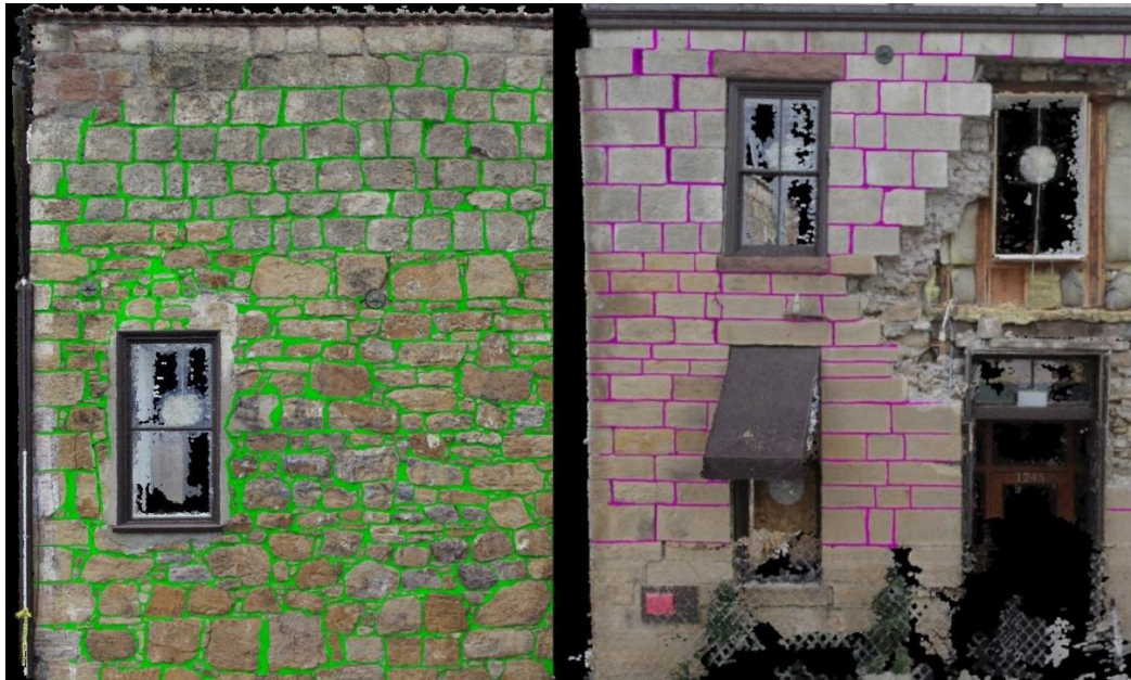
Figure 3.20 Manual ground truth annotation of mortar joints.
