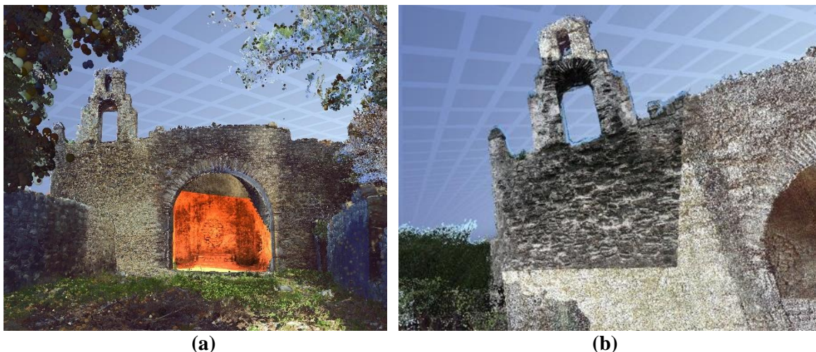
Figure 6.6 TLS points of the church used as a scaffold for aligned SfM images draped over in orange (a) and in photorealistic colors (b).
