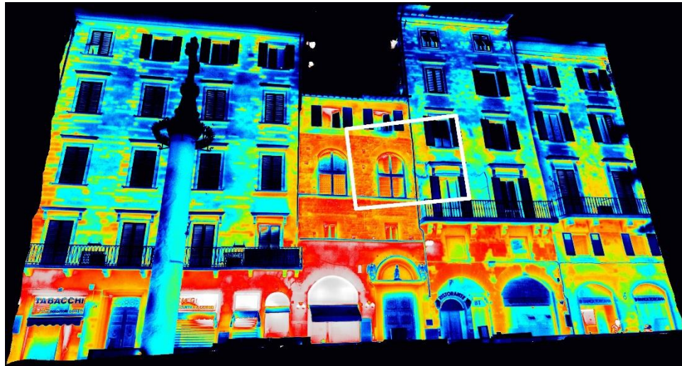
(b) Thermal image mosaic showing the entire building façade
