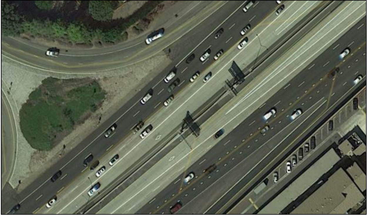
Figure 3: Limited Access Carpool Lane
