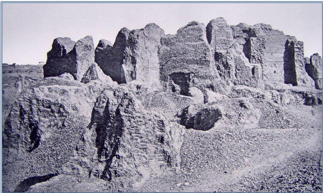
Figure 6. Remains of tower houses in Bubastis in 1880.
