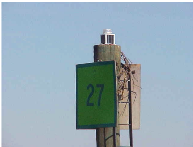
Figure 1 a. Pre-modified ATON night beacon with platform constructed during the late 1970s to encourage nesting and population resurgence.
