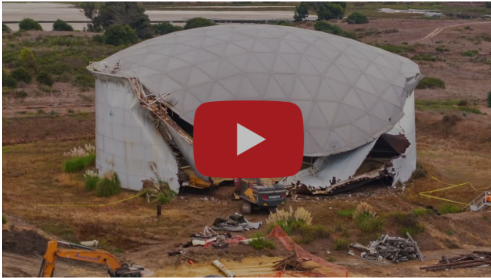
Deconstruction and grading at the EMT restoration site.
