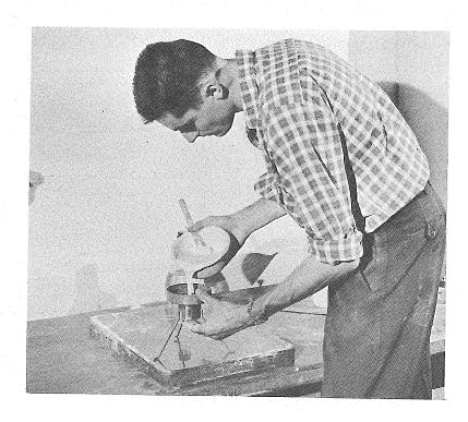
A - POURING PLASTER MIXTURE INTO CONSISTOMETER
