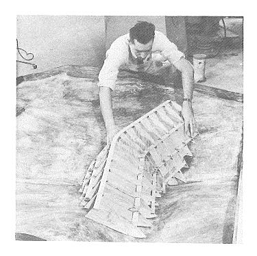
A - FRAMEWORK OF PLYWOOD TEMPLETS CONTROLS SHAPE OF PLUG
