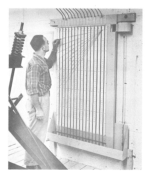
FIGURE 13 - MERCURY MANOMETER FOR CHECKING AIR BAG PRESSURE
