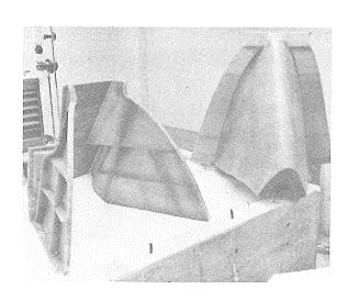
E - FIBERGLAS MOLDS EXPLODED
