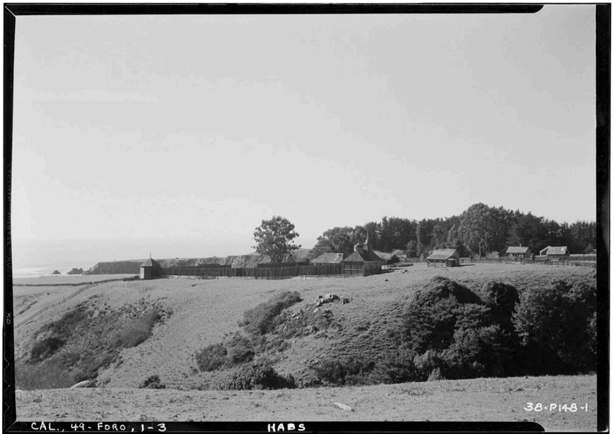
Figure 8. 10 Photograph by Roger Sturtevant for the Historic American Buildings Survey, 1934
