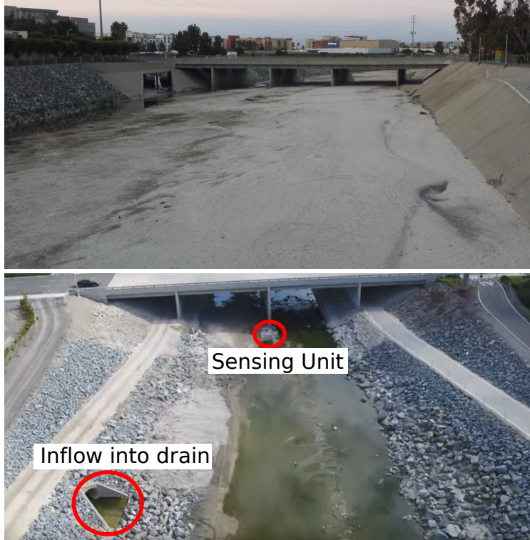
Figure 5.7: Our testbed in Orange County, USA: a storm drain and the locations of sensing units.
