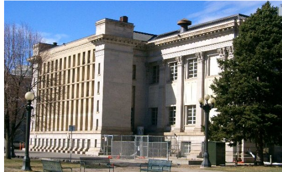
Figure 1-6. The 1910 Carnegie Library, located north across Civic Center Park from the DAM.
