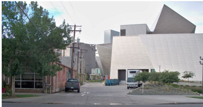
Figure 4-6. South end of the Hamilton Building. The 3 rd and 4 th floor on the north end are visible behind.
