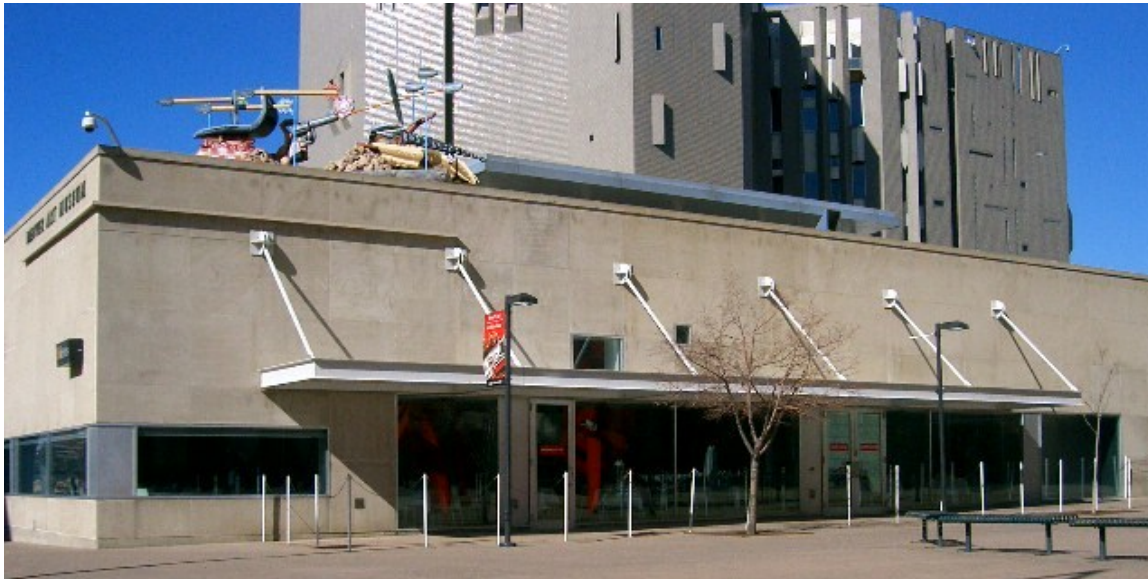
Figure 1-8. The South Wing, the Denver Art Museum's oldest existing building, and its first purpose-built building. It is now home to an upscale restaurant, Palettes.
