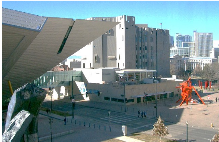
Figure 4-5. The north end of the Hamilton Building, towering over the 2-story Duncan Pavilion and gesturing towards the Pontifical and downtown.
