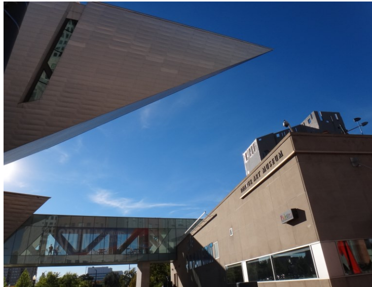
Figure 1-18. The Bridge connecting the second floor of the Hamilton Building to the Duncan Pavilion and the second floor of the North Building
