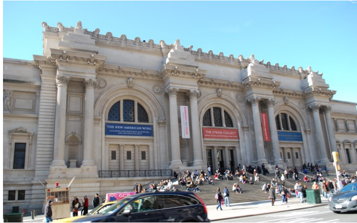
Figure 2-1. The Metropolitan Museum of Art, by Richard Morris Hunt in 1902, augmented a smaller building that faced the park. Note the stairs, the columns, and the decorative seals and busts, all signaling a building of importance.
