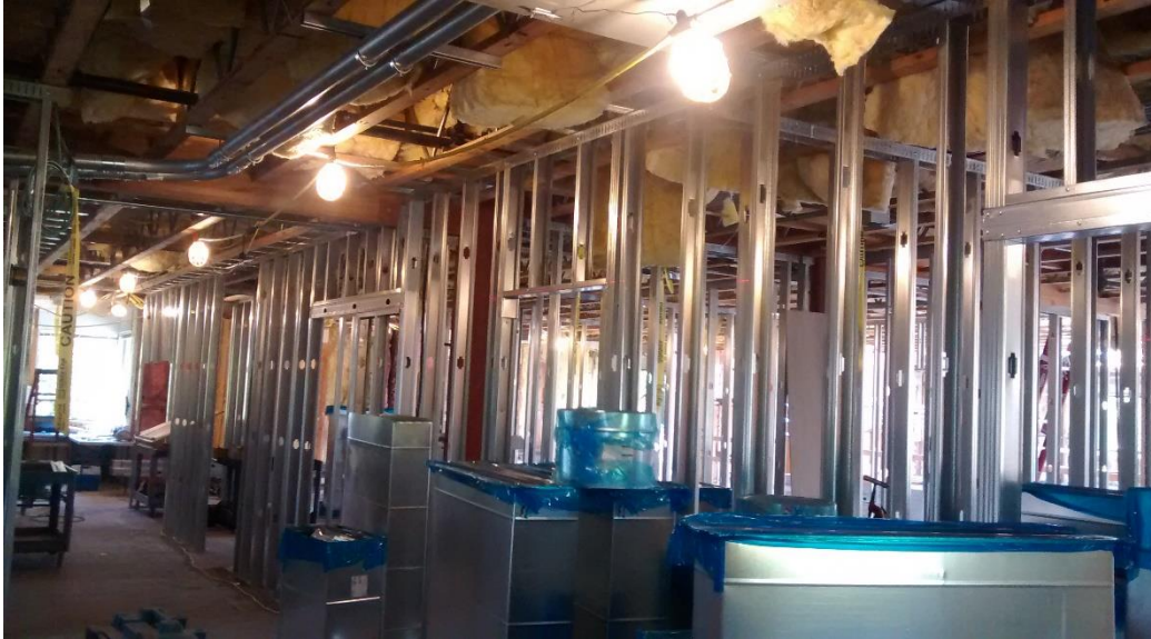
Figure 7-7 – Parallel fashion of work; wall framing, electrical, and duct install are nearly simultaneous due to crew sizes and space availability
