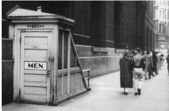
Figure 3: Public toilet stalls: The Rotary Club of Chicago's first public service project in 1907.
