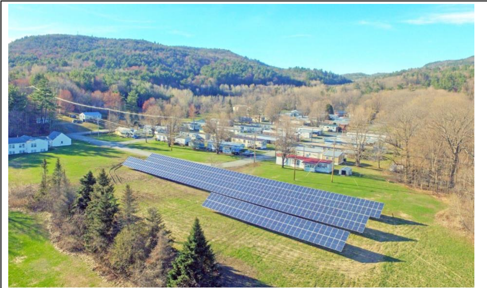
Figure 14: Mascoma Meadows MHC with solar installation
