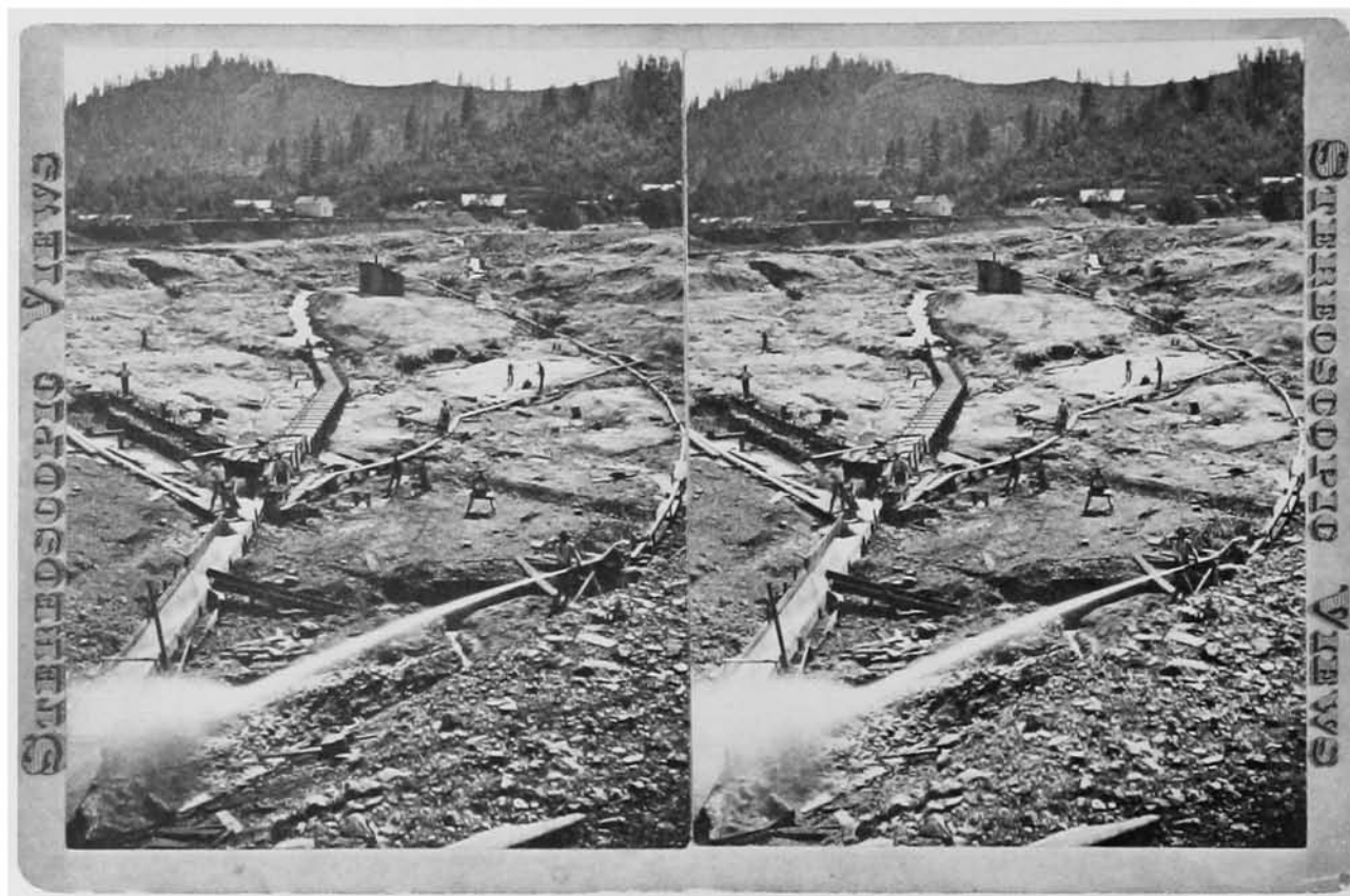
Plate 6. A Heller stereograph of hydraulic mining in the Oro Fino area.
