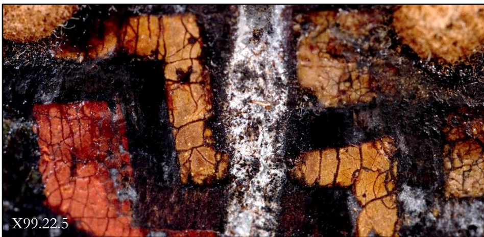
Fig. 21. Repair material on qero X99.22.5 showed organic fibers and a white efflorescence.
