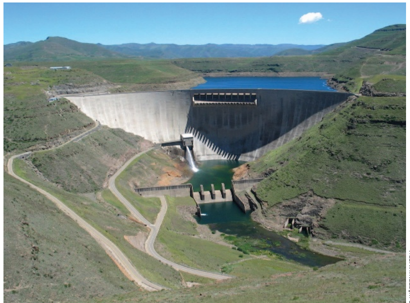
Katse Dam in Lesotho, Africa.
