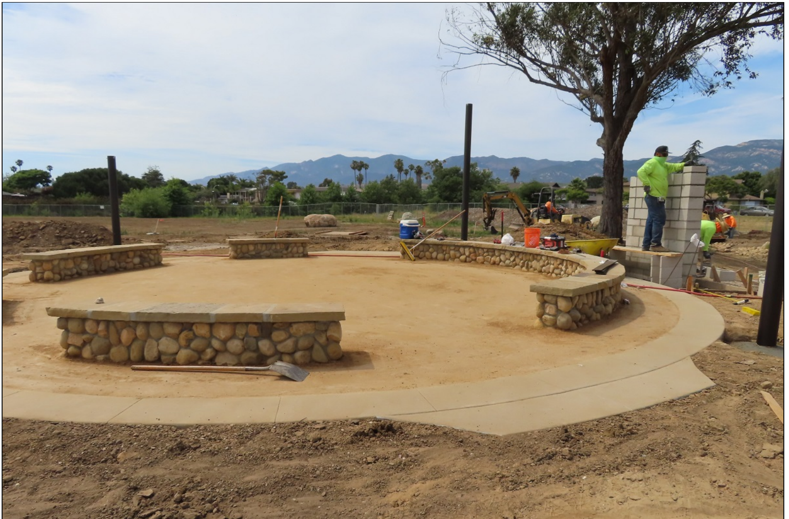
Construction of the NCOS Visitor Plaza is nearly complete.
