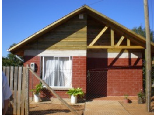
(b) site built masonry house
