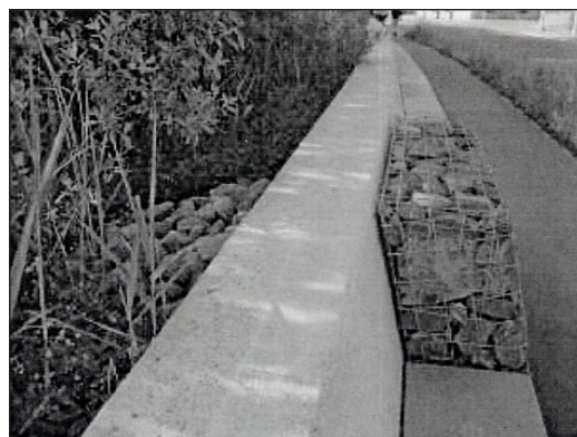
Figure 12. A pile of rocks (left side) or gabions filled with rocks (right side) can improve the permeability of a wall for small animals.
