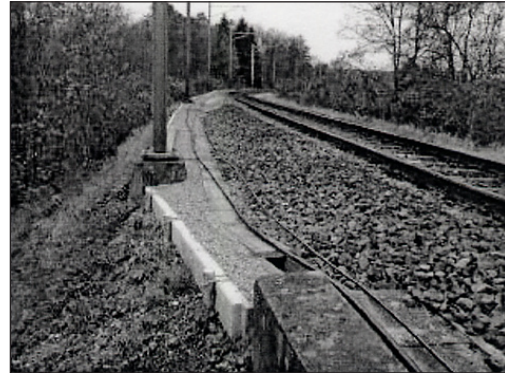
Figure 4. Even low retaining structures can be a strong barrier and prevent free crossing of a structure by small animals. (Photo courtesy to KARCH, Neuchâtel).
