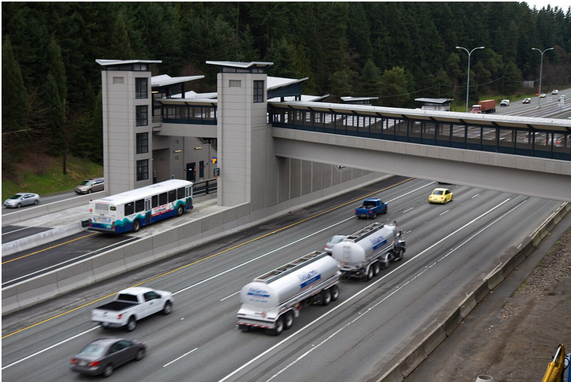
Figure 16. Inline Freeway Station Configuration — Seattle Region
