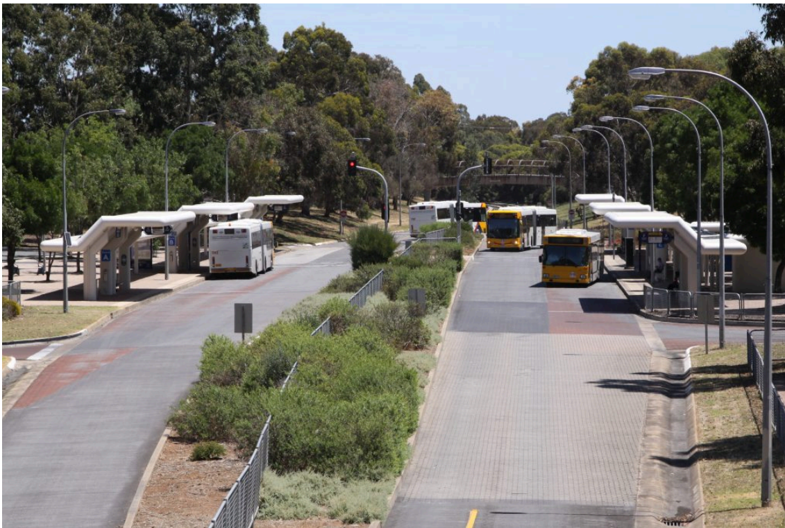
Figure 26. Guided Busway Guide-Rail and Interchange Station Configuration — O-Bahn
