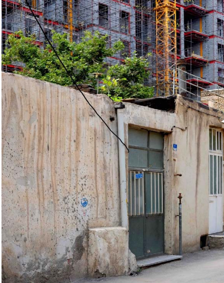
Figure 4.2: a high-rise being built in a narrow alley in Zafaraniye neighborhood. Source: photo taken by author, 2018
