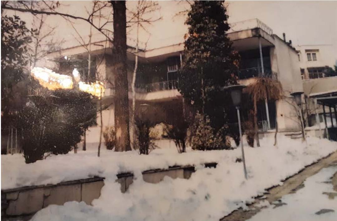
Figure 2.3: An old photo of Mina's family property before the demolition of their inherited villa, 1985. Source: courtesy of the interviewed family
