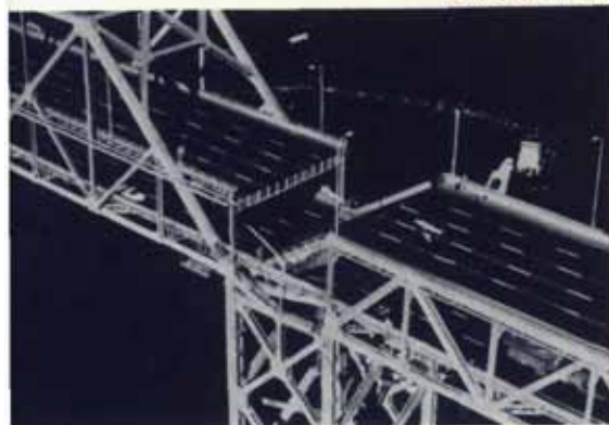
The section of the Bay Bridge upper deck fell when a bridge footing slipped out of place.
