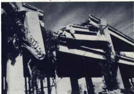
The double-decked section of I-880 in Oakland collapsed, crushing motorists on the lower deck.
