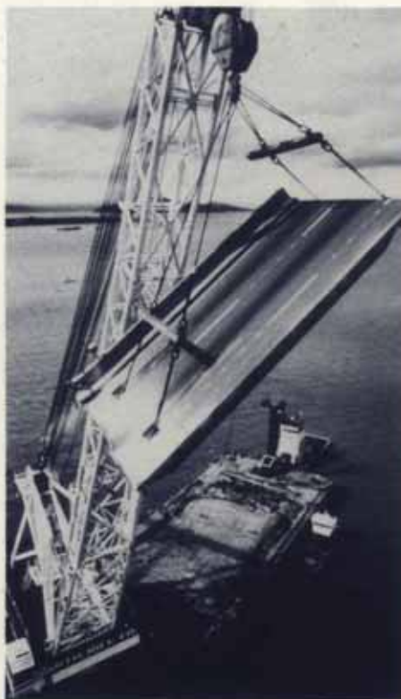
The replacement deck of the Bay Bridge being lowered into place, less than one month after the quake.
