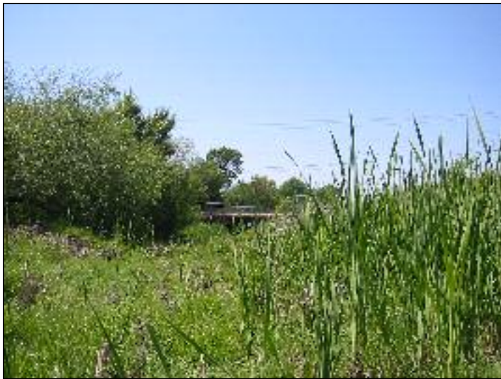
View of floodplain looking downstream. The Third St. bridge can be seen in the distance.
