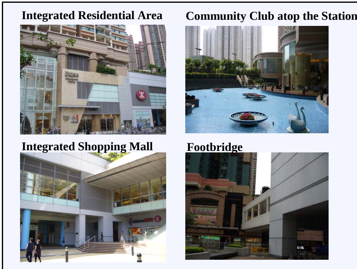
Photo 4.3. Hang Hau Station: Pedestrian Integration and Amenities
