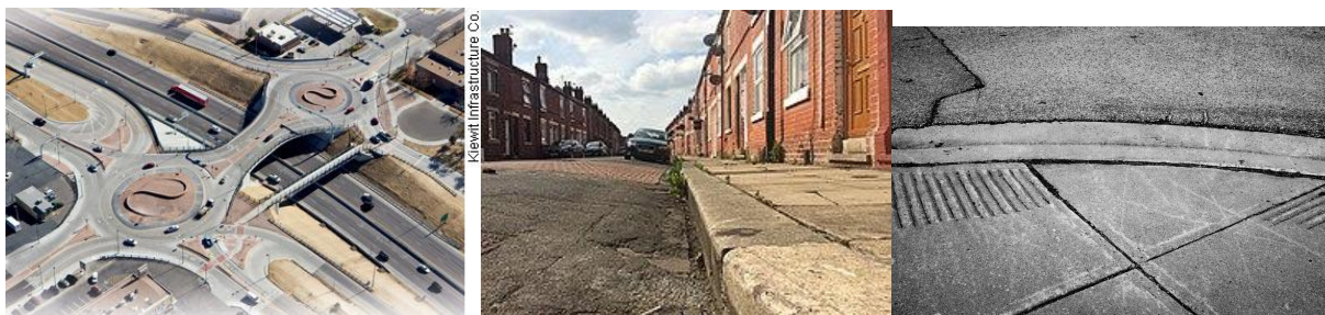
The geometric design of roads at different abstraction layers, left to right: highway interchange, road slope (to shed rainwater), and sidewalk-curb contraction joints (to minimize cracking).
