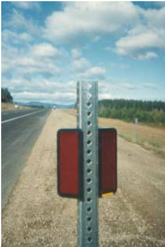
Fig. 1. Swarflex reflectors installed on a highway shoulder
