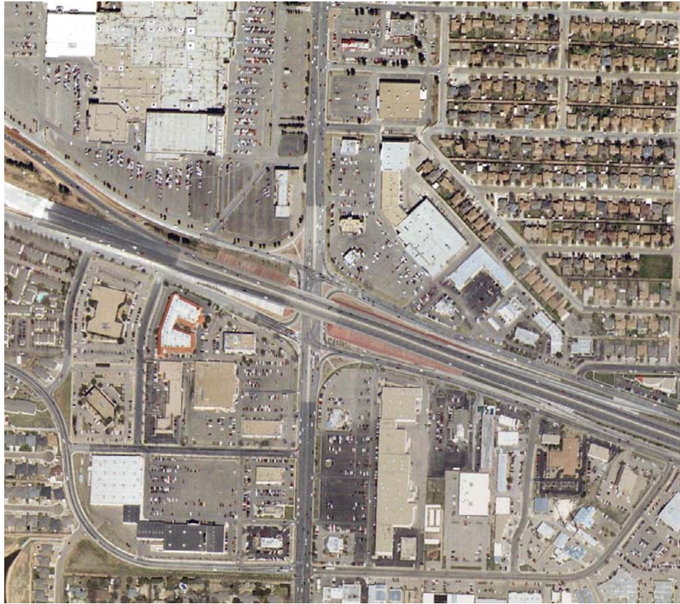
Figure 4.6 Aerial photo of the diamond Interchange
