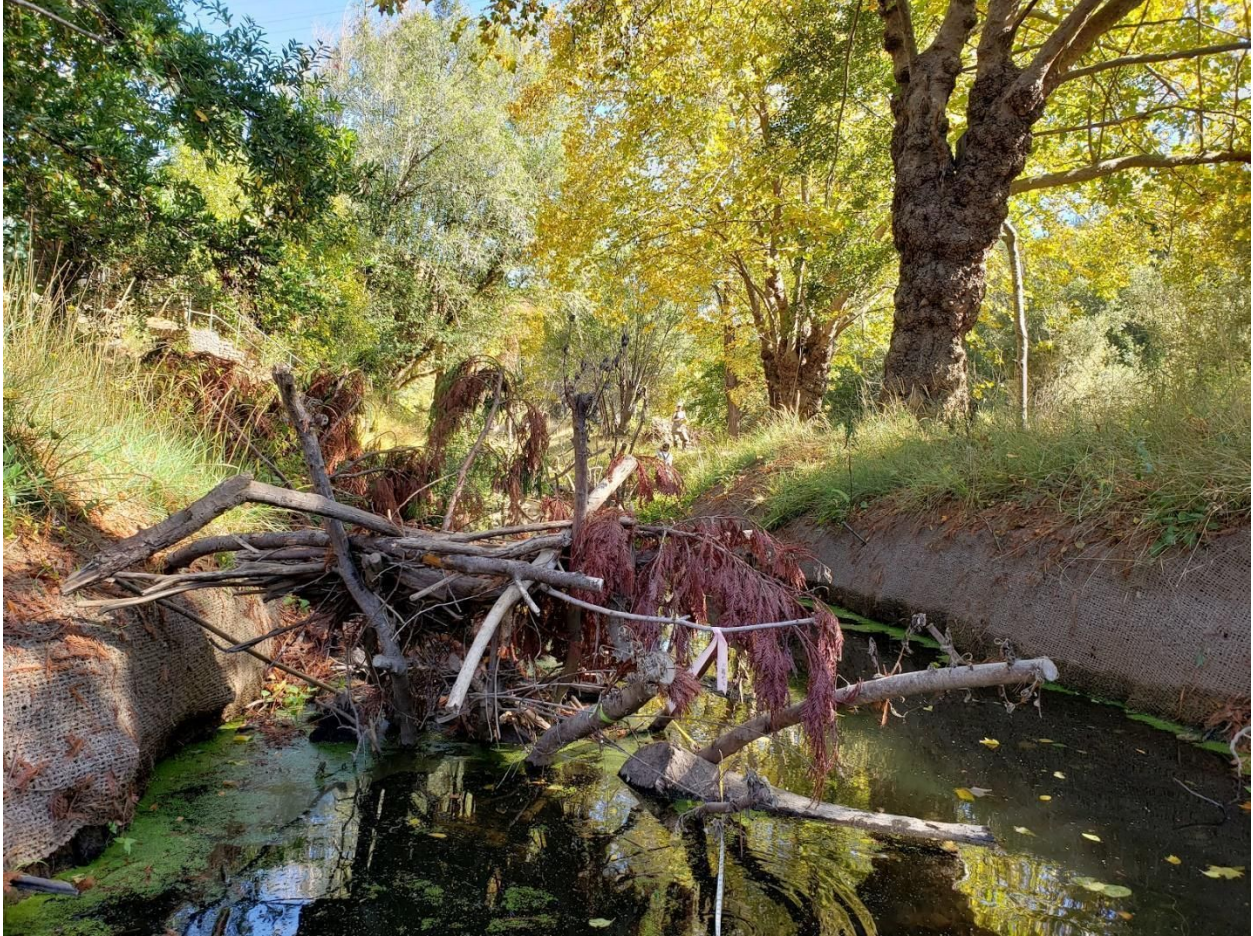
Figure 9: Constructed pile of large woody debris (and some non-transient woody debris) in the side channel. Constructed undercut banks covered in anti-erosion mesh are visible on the right and left banks.
