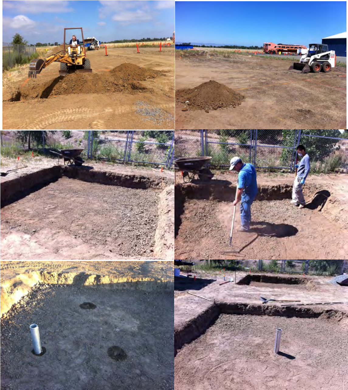
(a) Preparation of the subgrade layers.
