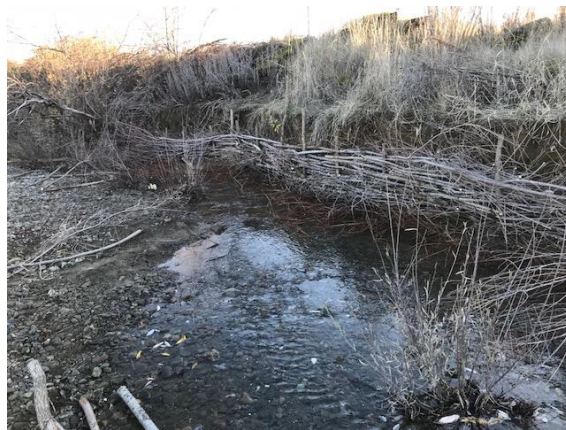
Figure 8. Willow wall installed in December 2017 for streambank stabilization 37
