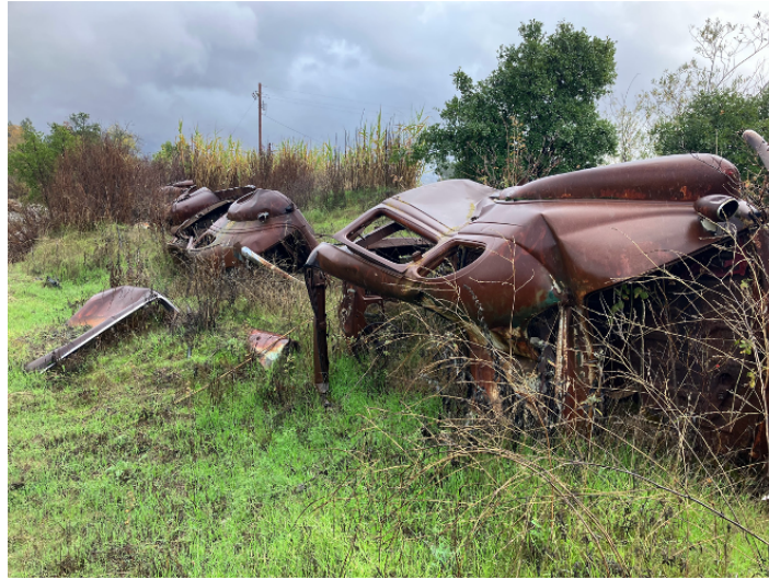
Figure 5. Wrecked cars as reinforcement on south bank
