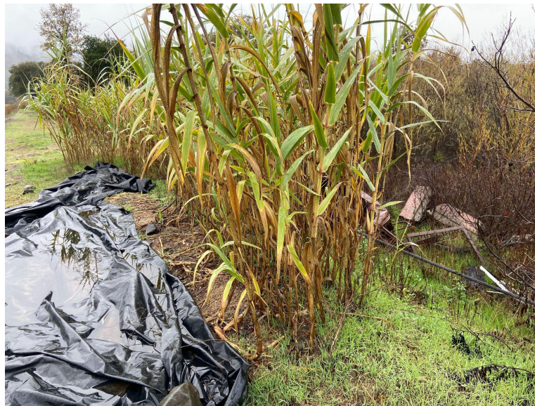
Figure 9. Arundo removal upstream of surveyed site, on south bank.
